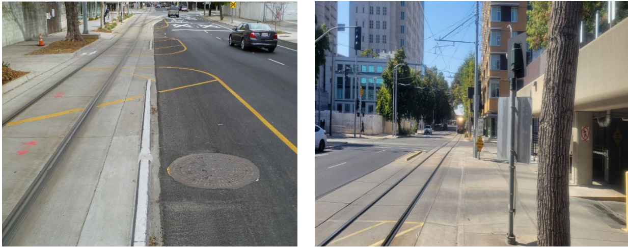
Figure 8 Photographs along H Street of Typical Light Rail Embedded Track on Concrete
